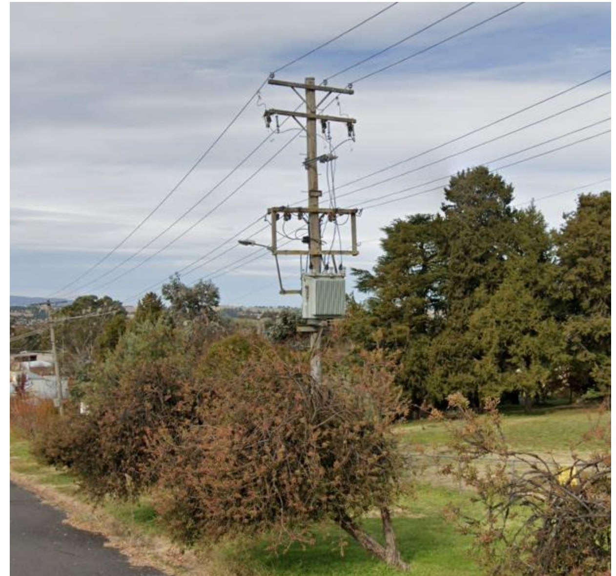
Figure 6: Existing Pole Mounted Substation (95-105)
